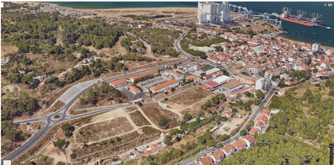
Figure 3: Aerial photograph of Trafaria with a view over the intervention area.
